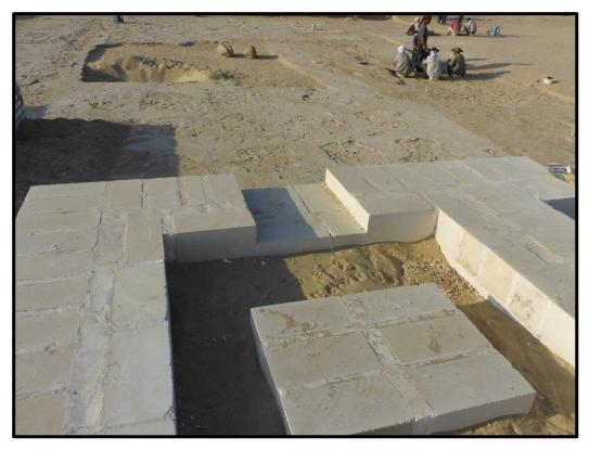
**Figure 9**: The rear part of the temple was filled with offering-tables, many of them inside individual small chambers. This offering-table has been completed, inside its chamber, as a sample of how the final scheme will look. View to the south.
