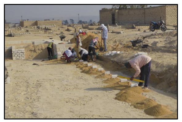
**Figure 6**: Builder Mohamed Shahata lays a preliminary line of blocks along a string guideline and checks that all follow a horizontal plane. The blocks rest on piles of sand which protect the underlying foundations and allow for easy adjustment of each block.
